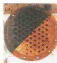
HEAT EXCHANGER TUBE CLEANING
