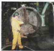
EVAPORATOR TUBE CLEANING
