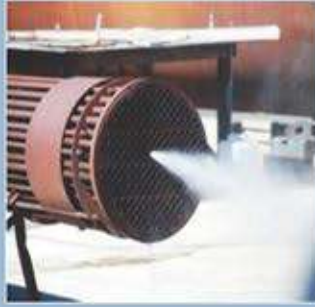
Internal Tube Cleaning
