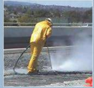
Concrete Removal
