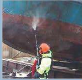
Ship Hull Cleaning
